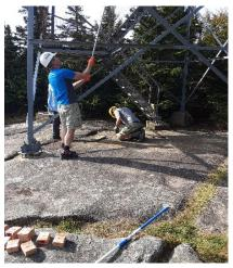
**St. Regis:** The crew at St. Regis has continued to be very busy with routine maintenance and repairs at the fire tower despite the late calendar date. The crew has been painting, making certain there is a protective layer between the steel and the pressure treated lumber and also cleaning out the leg brackets. Cooler weather does not stand in the way of this ambitious group of volunteers! Thanks for all of your work!
